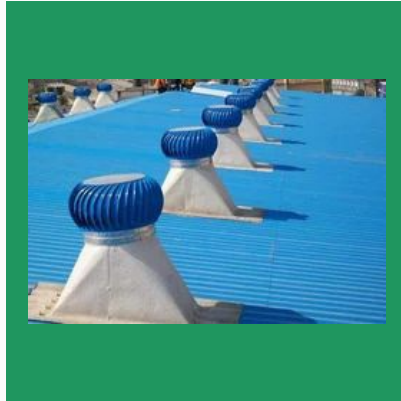
Automatic Turbo Ventilator
