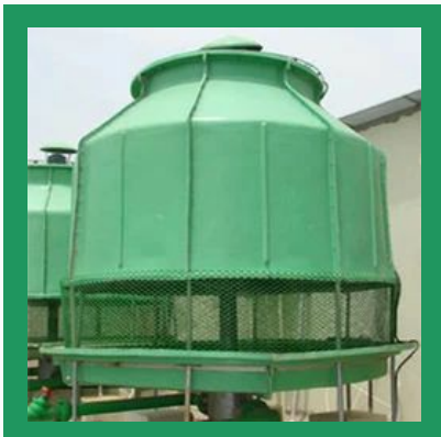
FRP Induced Draft Cooling Tower
